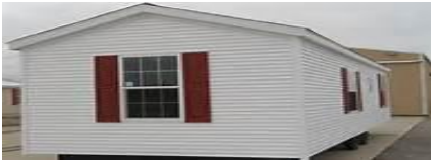
This view IS NOT acceptable facing internal road
